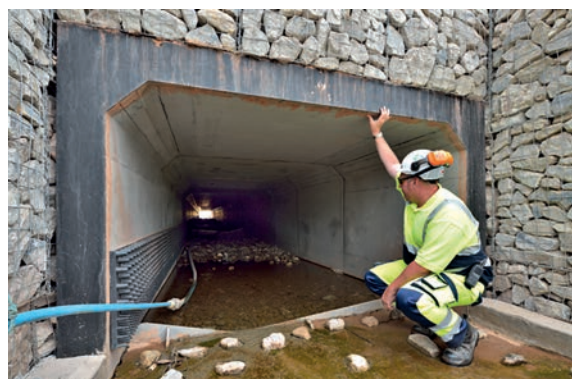
Environmental work onsite: box culvert with eel pass
